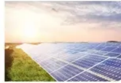
Energy Storage System
